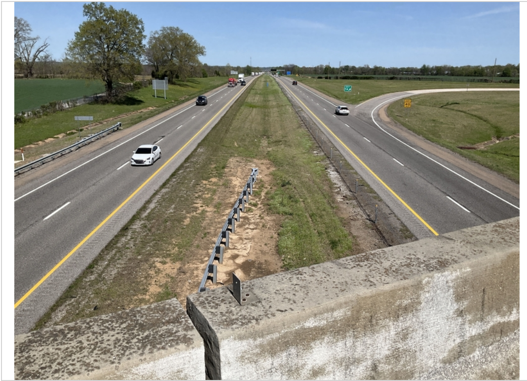
Roadway beneath bridge (I40) looking right off bridge
