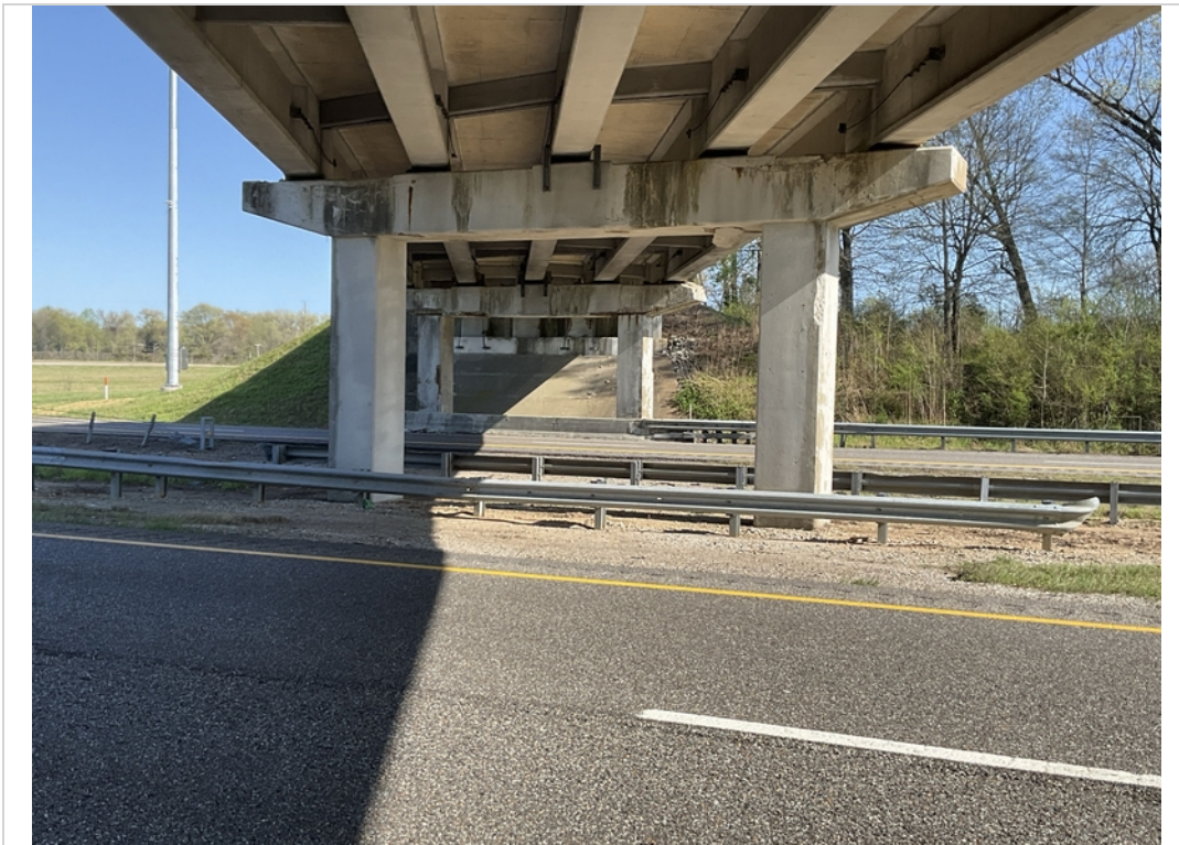
Bent 2 back face (Span 3 side)
