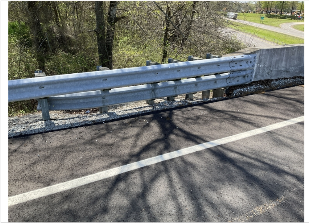
Approach 1, left transition with rub rail and rails bolted to barrier
