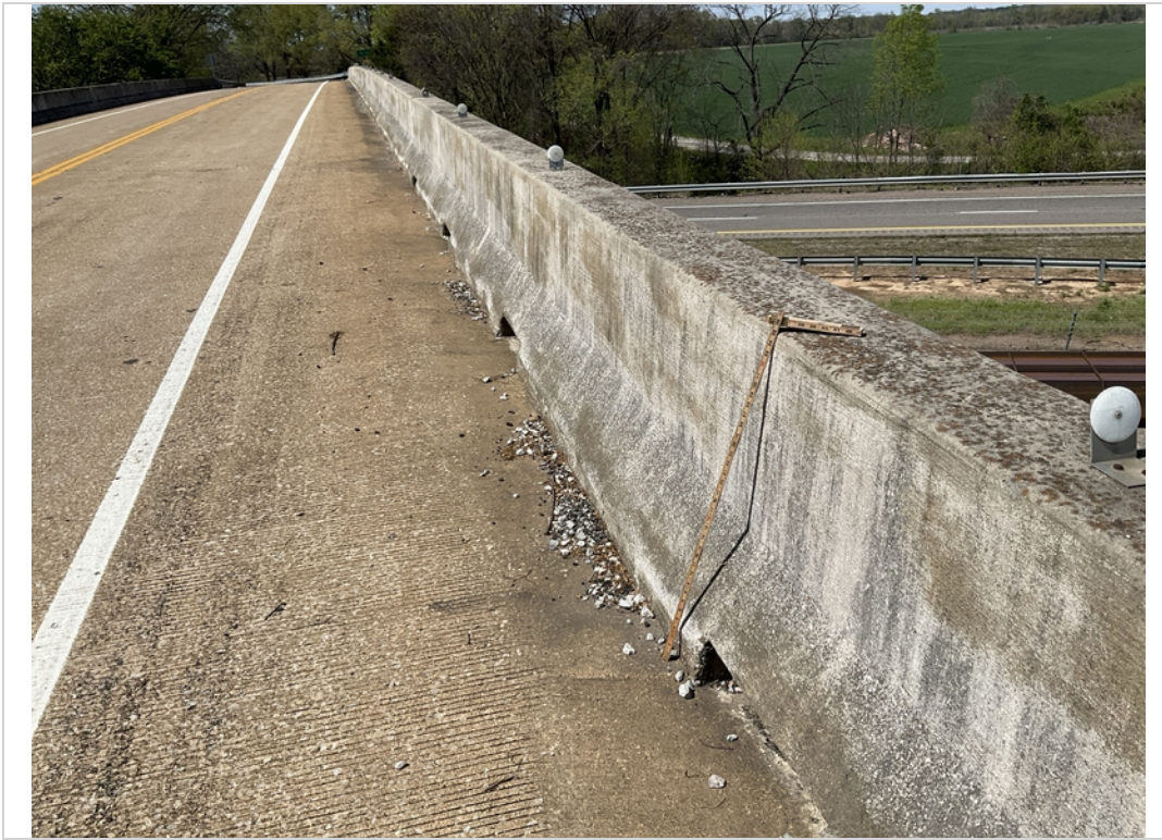
Span 1, right bridge rail, concrete safety shape. Spans 1 and 4 have drains through barrier bases
