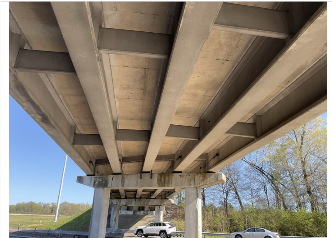
Span 3 deck underside and superstructure, looking back
