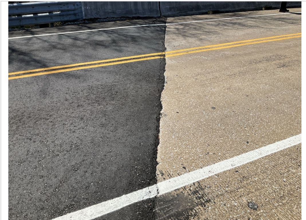
Pavement match line over Abutment 1 from asphalt approach to concrete bridge deck
