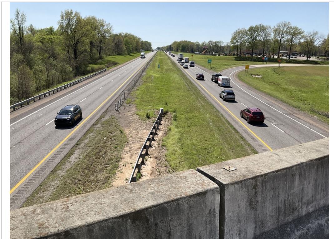
Roadway beneath bridge (I40) looking left off bridge
