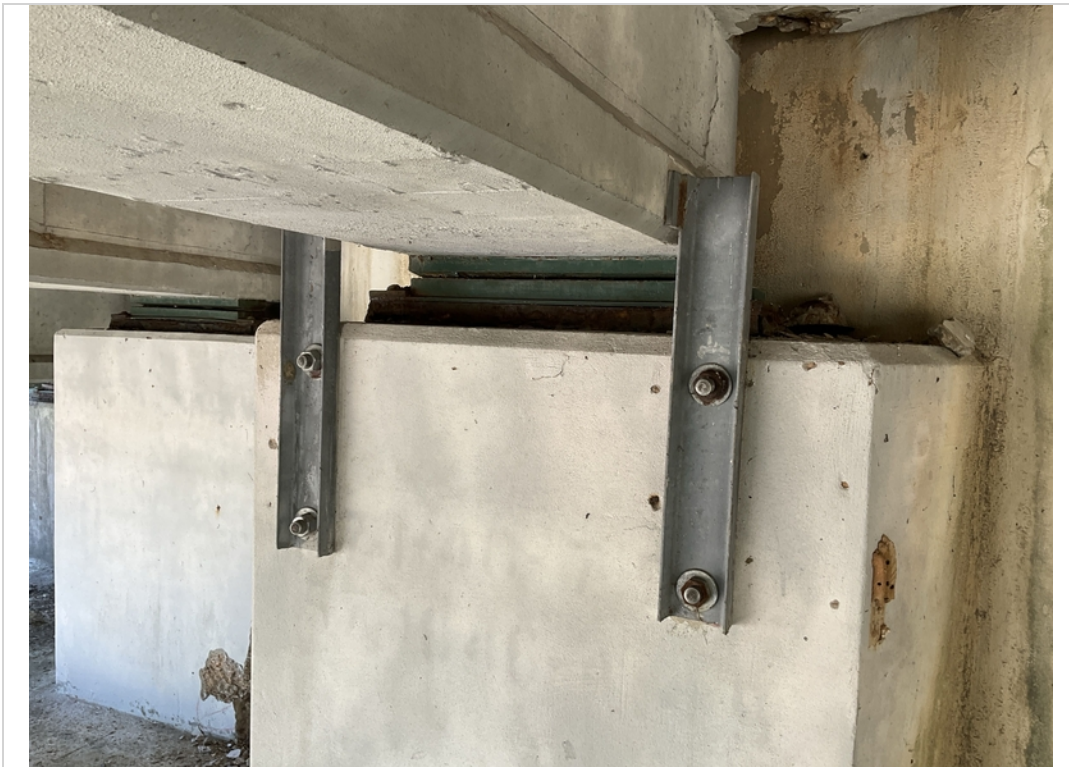
Span 1, abutment 1, Beam C, lateral keepers installed for beam alignment
