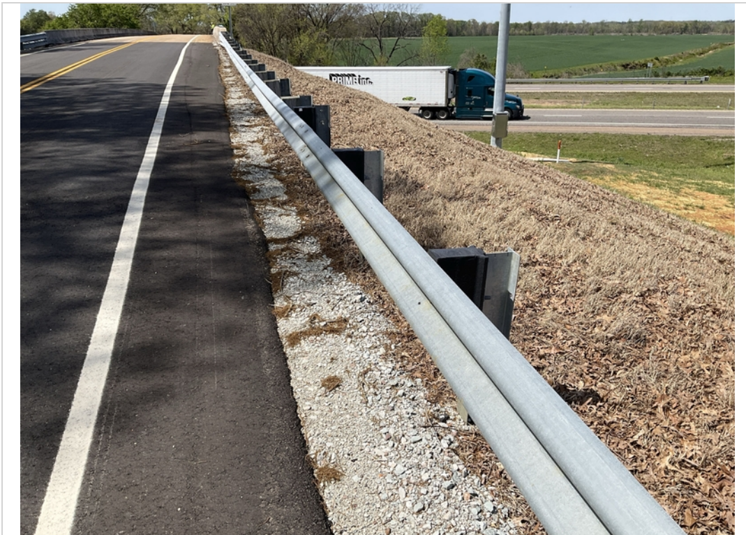
Approach 1 right guiderail with plastic and timber offset blocks
