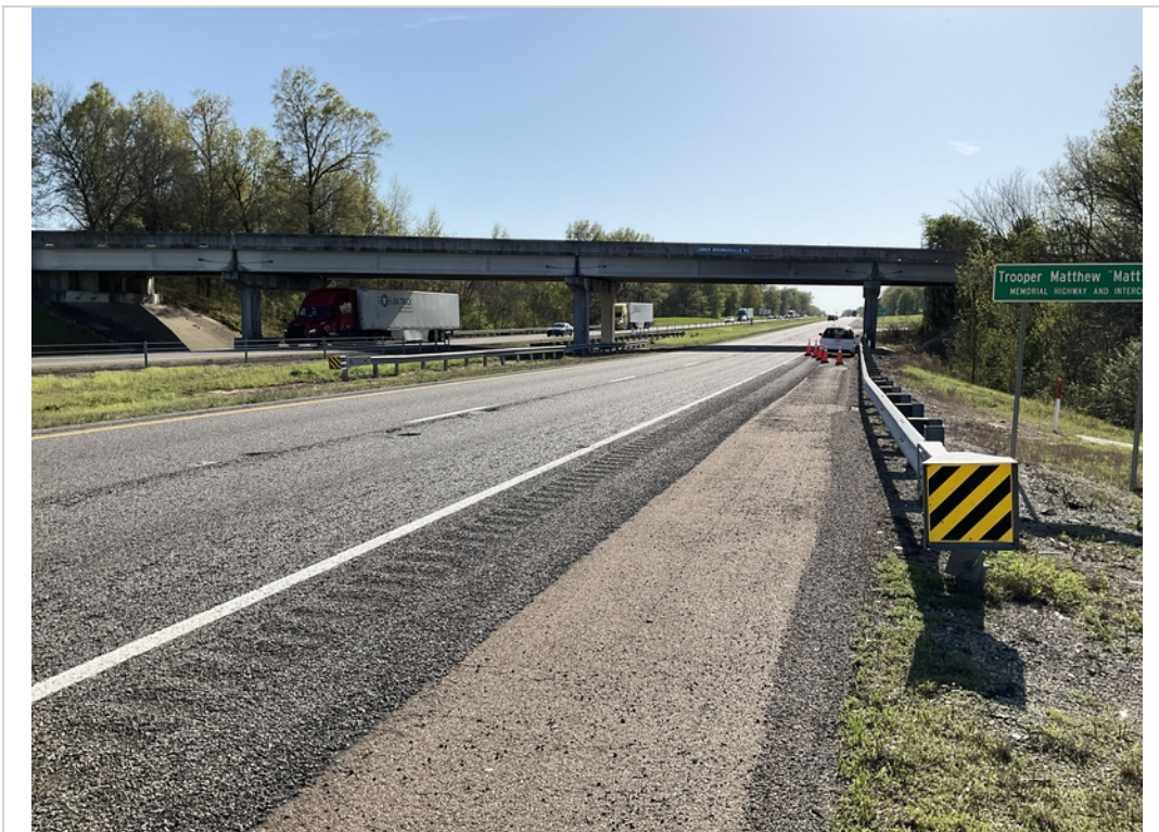
Right elevation looking left
