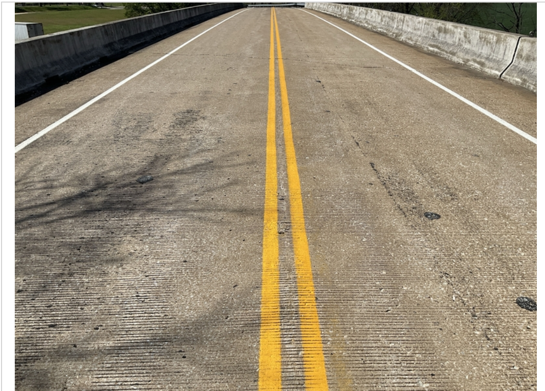
Span 1 bridge deck looking ahead
