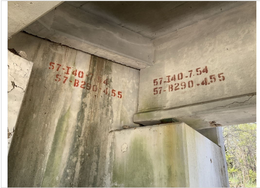
Abutment 1 and Beam A, bridge ID painted on backwall and right side of beam
