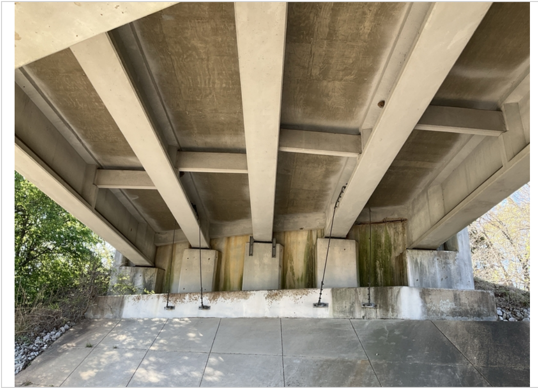
Span 4 deck underside and superstructure, looking ahead
