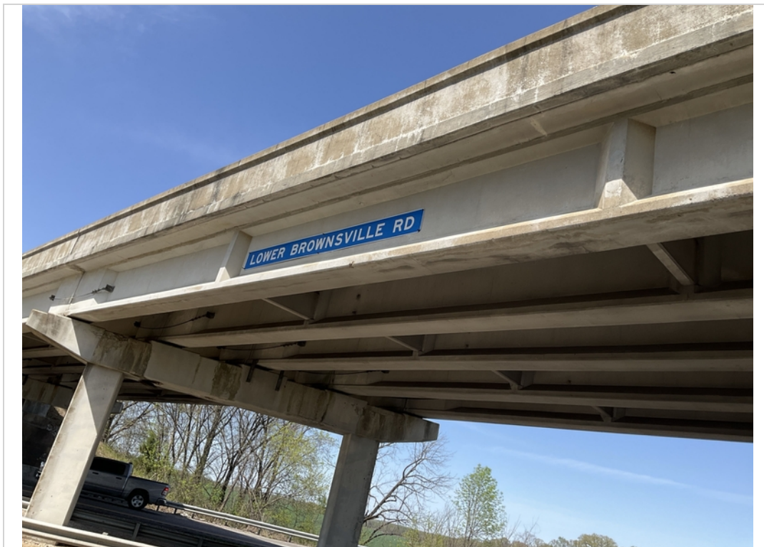
Sign attached to Beam A, Span 2
