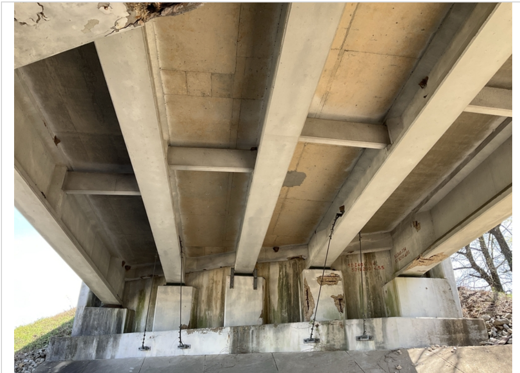
Span 1 deck underside and superstructure, looking back
