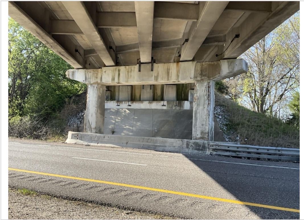
Bent 3, front face (Span 3)
