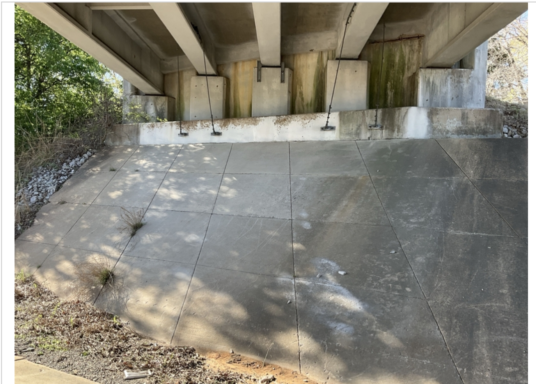
Abutment 2 with concrete slope protection with areas of adjacent stone/rip-rap protection along the edges.
