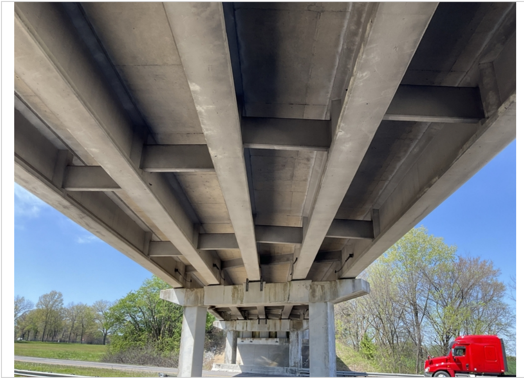
Span 2, deck underside and superstructure, looking ahead
