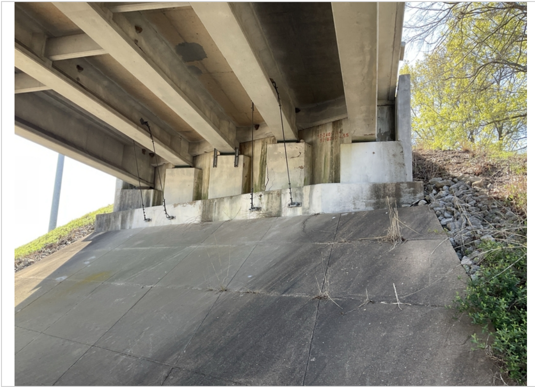
Abutment 1 with concrete slope paving and adjacent stone/rip-rap protection along the edges.
