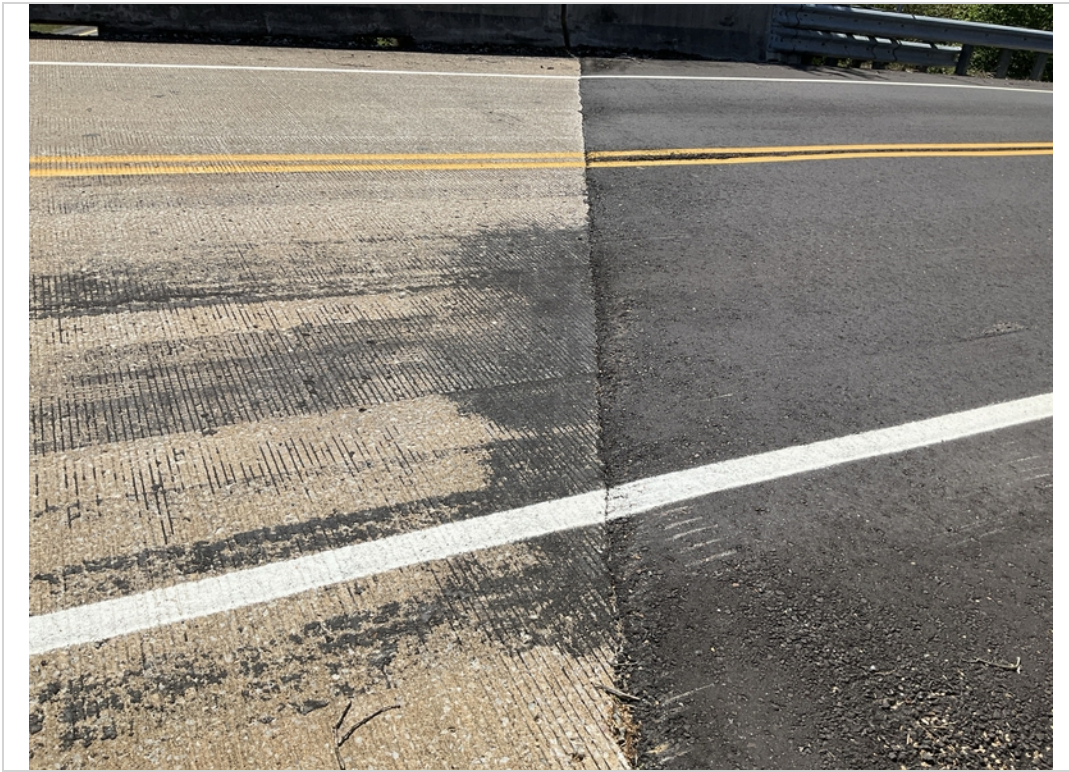
Pavement match line over Abutment 2 from asphalt approach to concrete bridge deck
